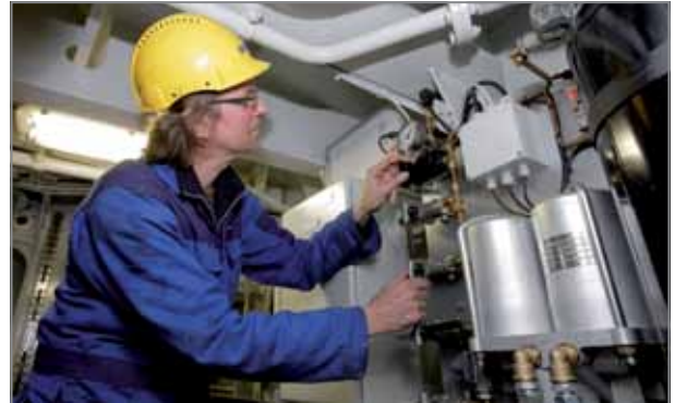
EXECUTED BY A DAMEN SERVICE ENGINEER
