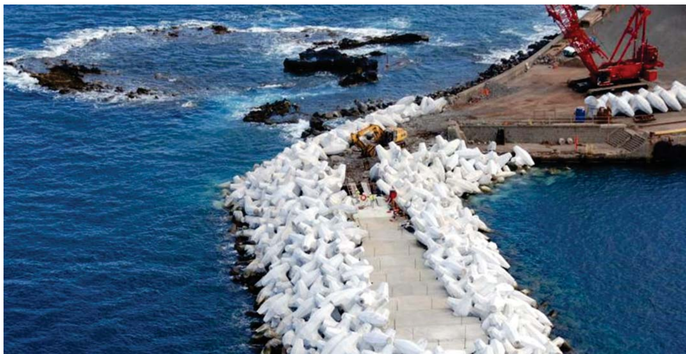
BREAKWATER (CONCRETE ARMOUR) EXECUTIONAL WORKS
