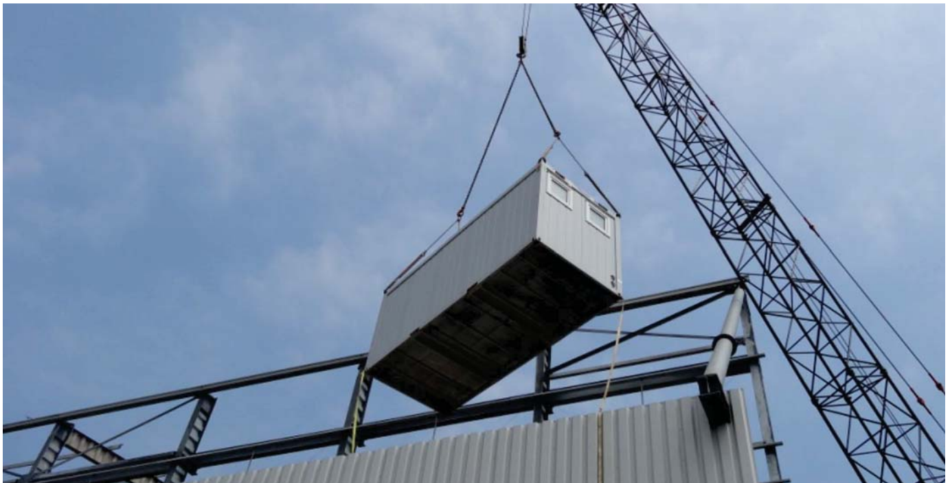
LIFTED WITH A MOBILE CRANE
