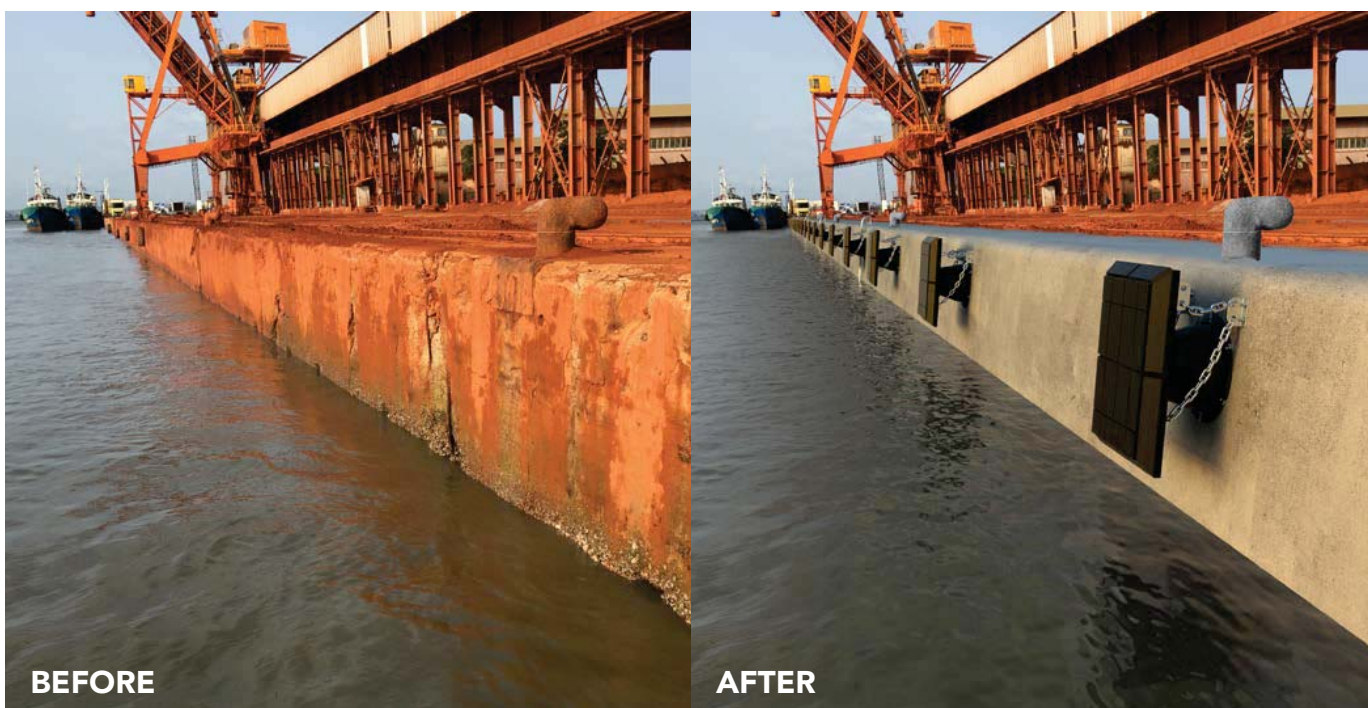
REHABILITATION OF EXISTING QUAY WALL
