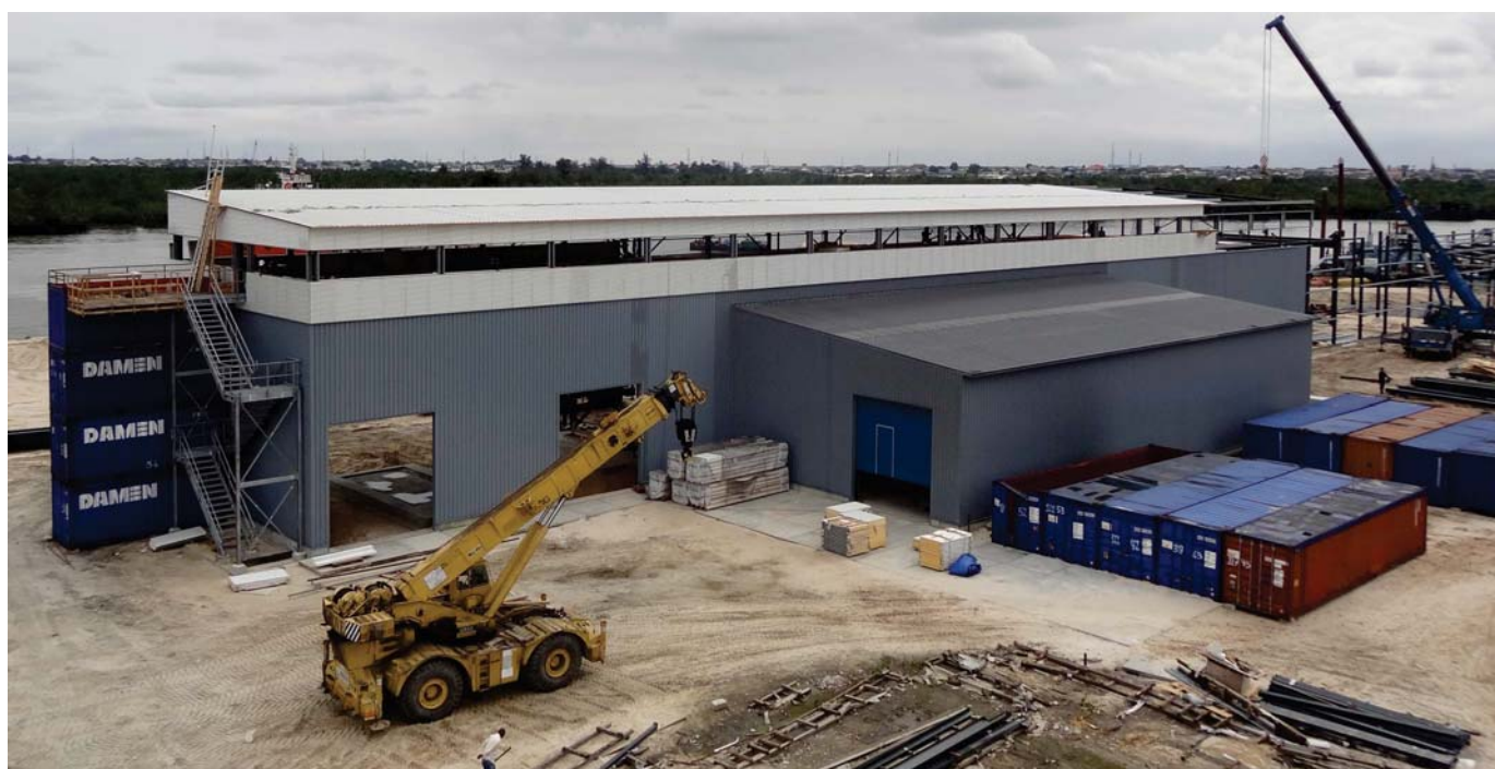
REPAIR FACILITY EXECUTIONAL WORKS
