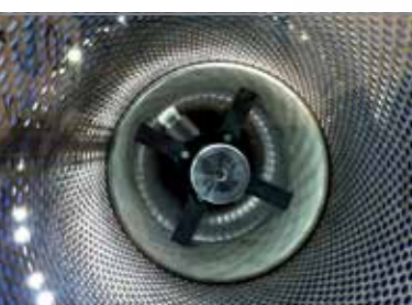
ONE STOP RETROFIT SERVICE
